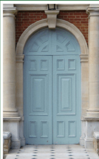
The repair and restoration of the south porch
